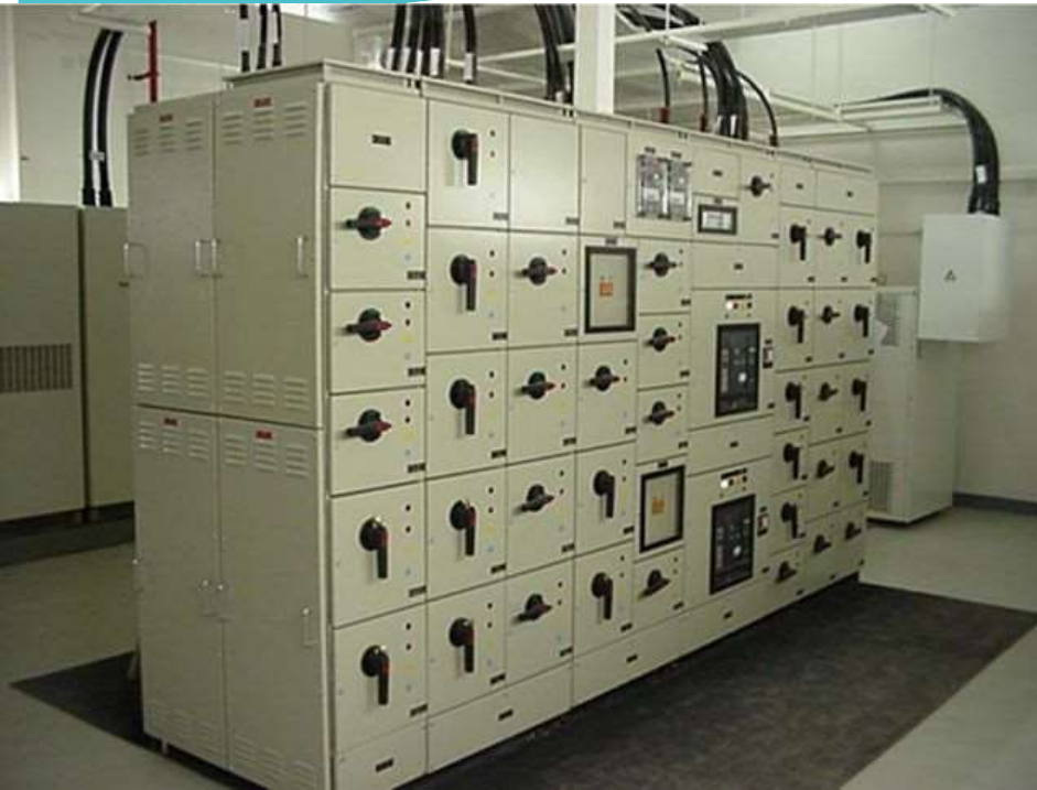
电力配线柜 Distribution Cubicle
